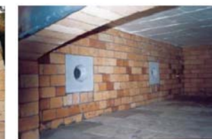
Figure 2b. Refractory walls of a furnace interior with burner blocks (BEE, 2005)
